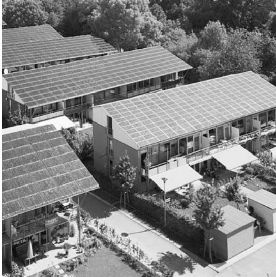
FIGURE 1. The solar estate, “ Solarsiedlung Freiburg am Schlierberg. ” 59 plus-energy terrace houses, nine of them on the flat roof an office block. Source: Büro Disch.
